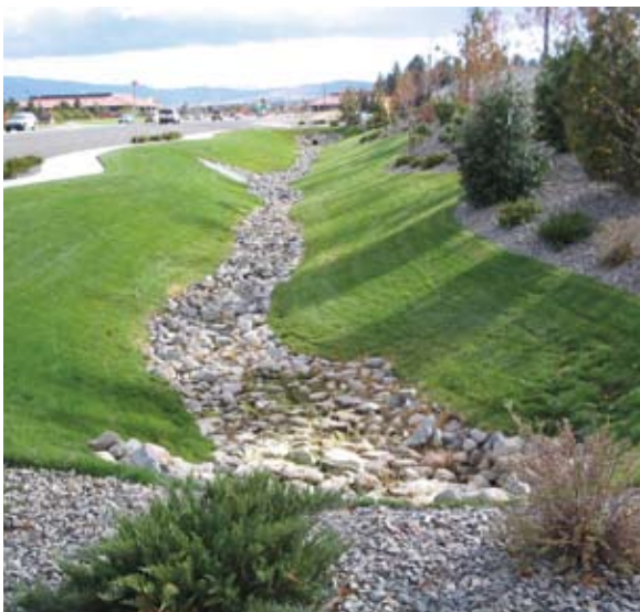
This large grassed swale can infiltrate and filter runoff. It is easier to clean sediment out of basins and swales than from underground infiltration systems.
