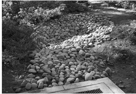
The overflow spillway of this infiltration basin is at the low point under the mature shrub.
