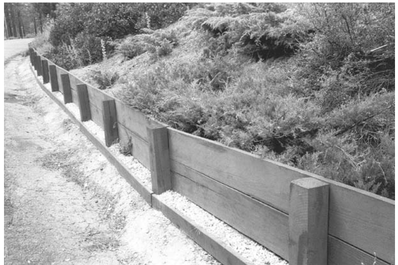
Other common methods of slope stabilization include wood retaining walls, interlocking concrete blocks and riprap.
