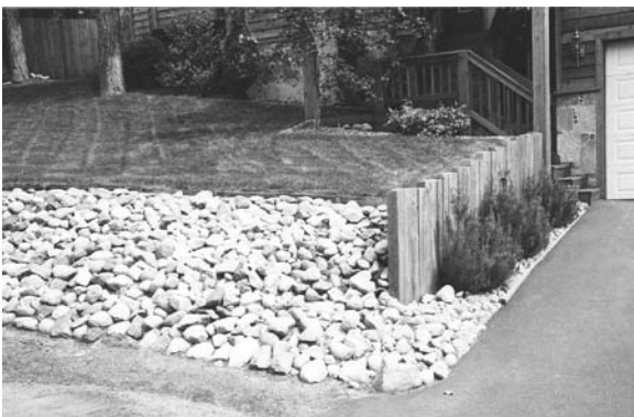
Other common methods of slope stabilization include wood retaining walls, interlocking concrete blocks and riprap.
