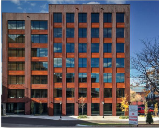
The T3 building in Minneapolis, Minnesota, USA (Brownell, 2016)
