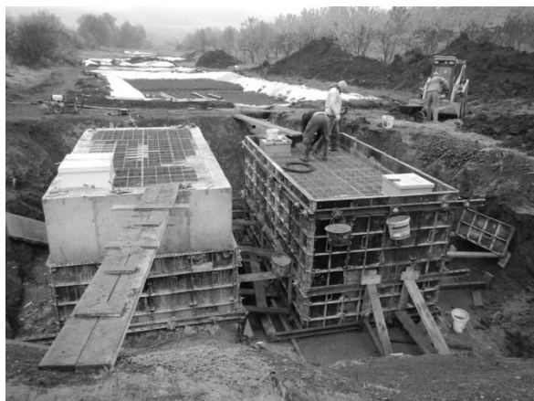
Fig. 1. CW in construction 2012.
