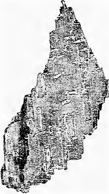
FIG. 290.— Agaricus adiposus . Destruction of Fir-wood. The deeply-corroded cross-fissures contain white mycelium; the remainder of the wood is yellow. (v. Tubeuf phot.)
