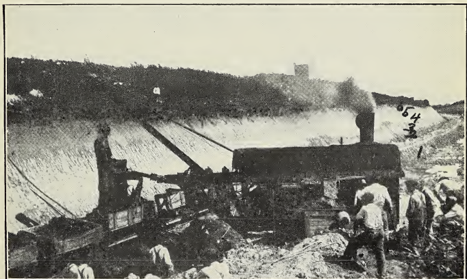
A second view of the cut east of Sandyville.
