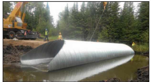
Mullett Creek new culvert installment
