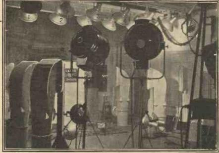
Groups of up to six persons are scanned by mechanical means in the French television studio seen here. Special ducts for cooling air are used to counteract the heat dissipated by the 40 kws. of lighting employed.
