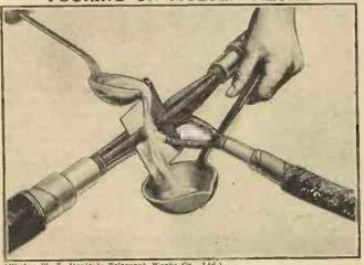
(Photo: W. T. Henley's Telegraph Works Co., Ltd.) How copper conductors are joined in cable work.
