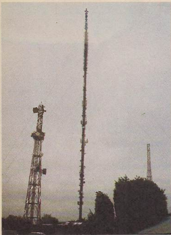
A recent shot of the Oxford (Beckley) TV transmitting mast, taken by Ian Beckett (Buckingham). Note the profusion of dishes and mobile communications aeriols bolted to the sides of the lattice structure.
