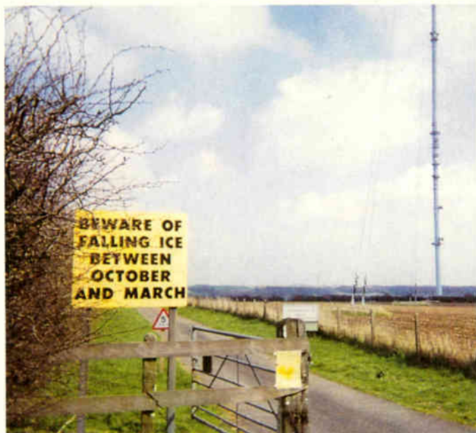
Access road to the current Belmont transmitter mast. Note the ice in winter warning.
