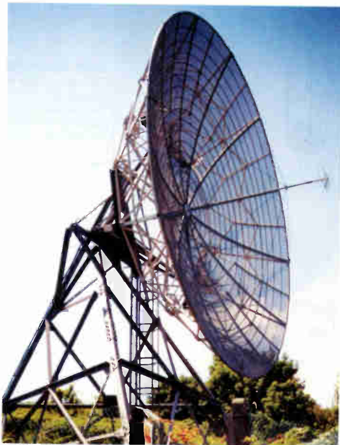
The 30ft parabolic dish, now disused, that was originally installed at Braye Bay, Alderney for reception from Stockland Hill.
