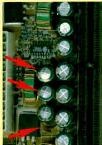
Photo 1: A group of faulty PC motherboard electrolytic capacitors.
