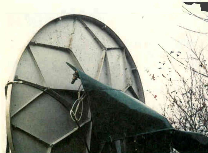
Dirt on the rear side of the dish. Note PVC covers used to protect the actuator arm.
