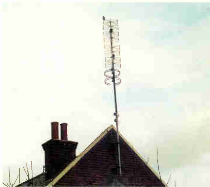
Stacked bow-tie aerials with, below, a couple of FM loops. Seen at Arundel in West Sussex.
