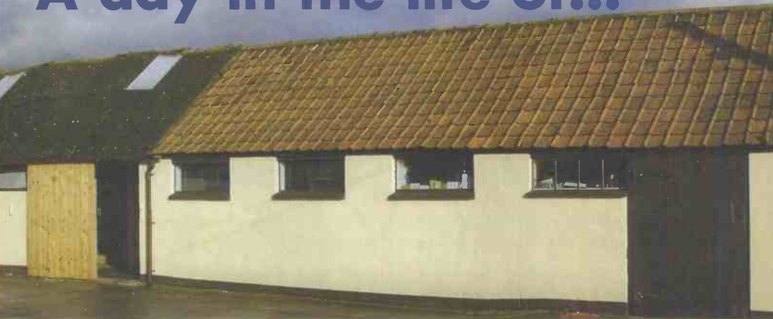
The premises of Dolman Electronics, converted from a milking parlour
