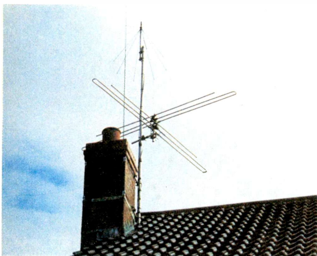
The omnidirectional, wideband crossed dipole aerial system described in the text, for Band I operation.
