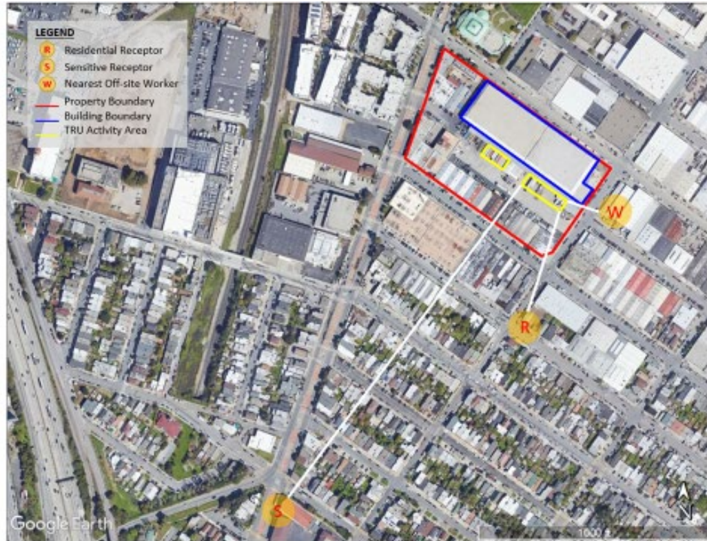
Figure II.G.1. Aerial Image and Spatial Analysis of a California Cold Storage Warehouse
