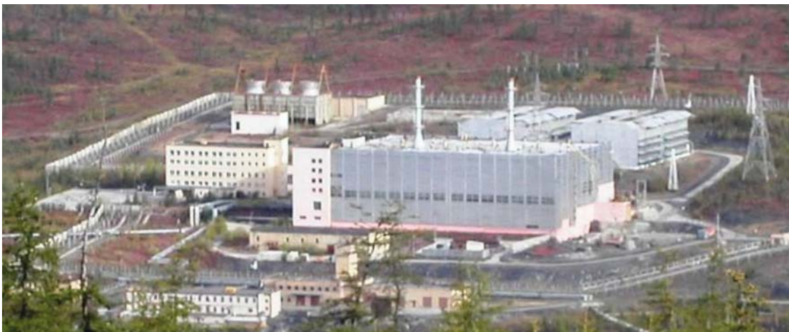
FIG. 43. Picture of Bilibino Nuclear power plant operating with dry cooling system.
