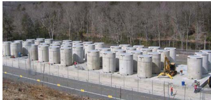
FIG. 7. ISFSI Site in Haddam, Connecticut with 43 dry storage dual purpose casks.
