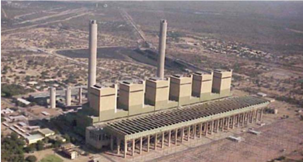
FIG. 41. Matimba, 6 \times 665 MW(e) coal power station.
