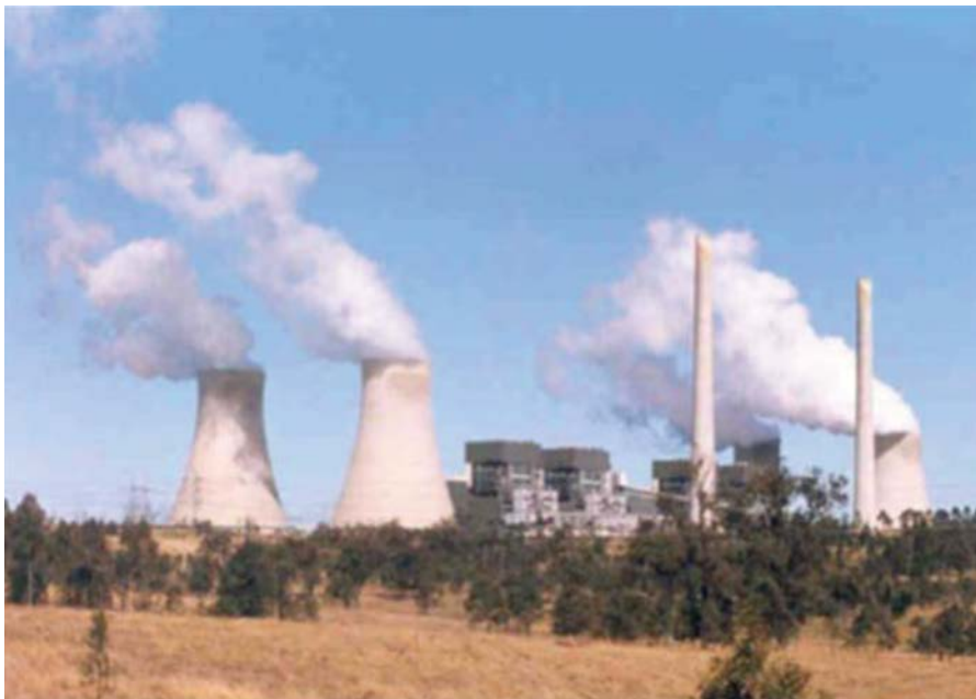
FIG. 39. Bayswater power station (4 × 660 MW) New South Wales, featuring natural draft evaporative cooling tower.
