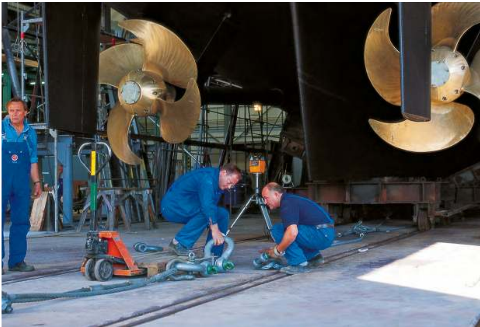
A great moment approaches: taking out of dock after a construction phase of several years
