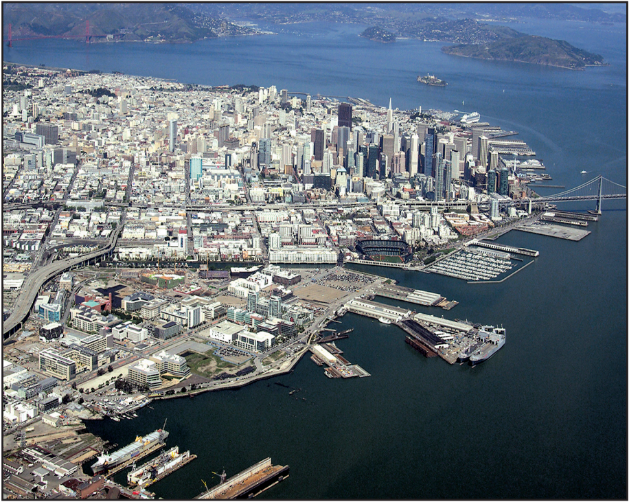
Photo courtesy of the Port of San Francisco
