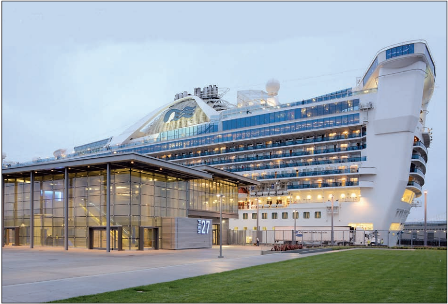
James R. Herman cruise terminal at PIER 27, courtesy of Port of San Francisco
