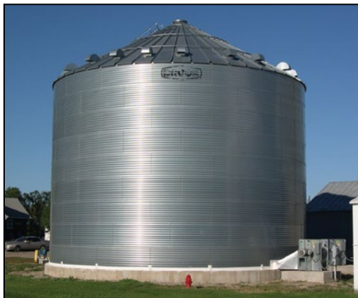
Figure 129. Structures adequate to store other grains are adequate for sunflower.
