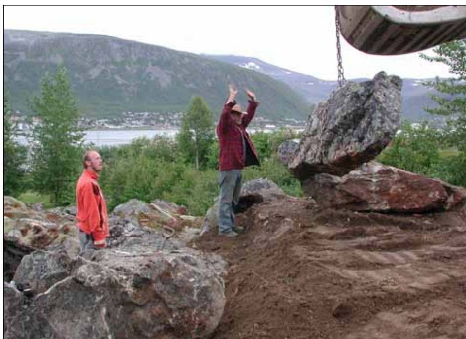
Steps in construction work (photos by Arve Elvebakk)
