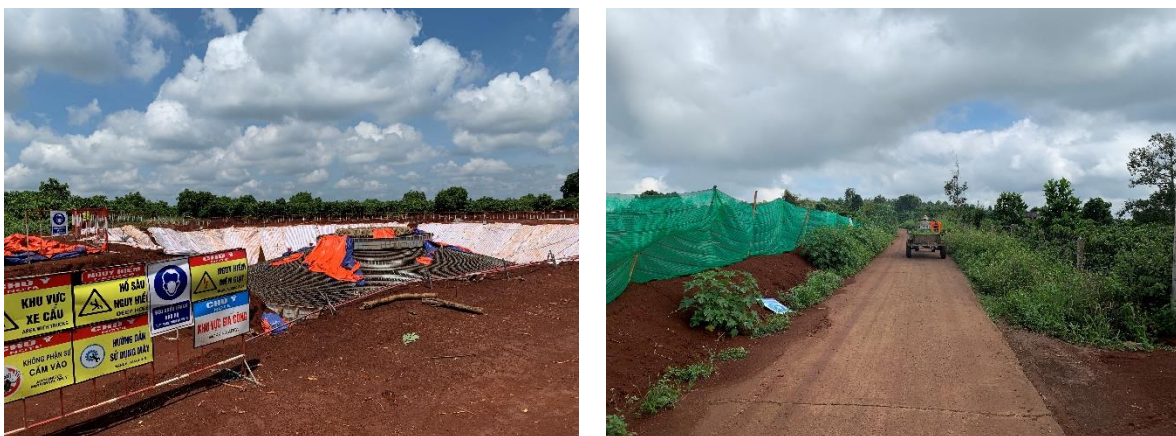
Source: ERM's site visit in May 2021
