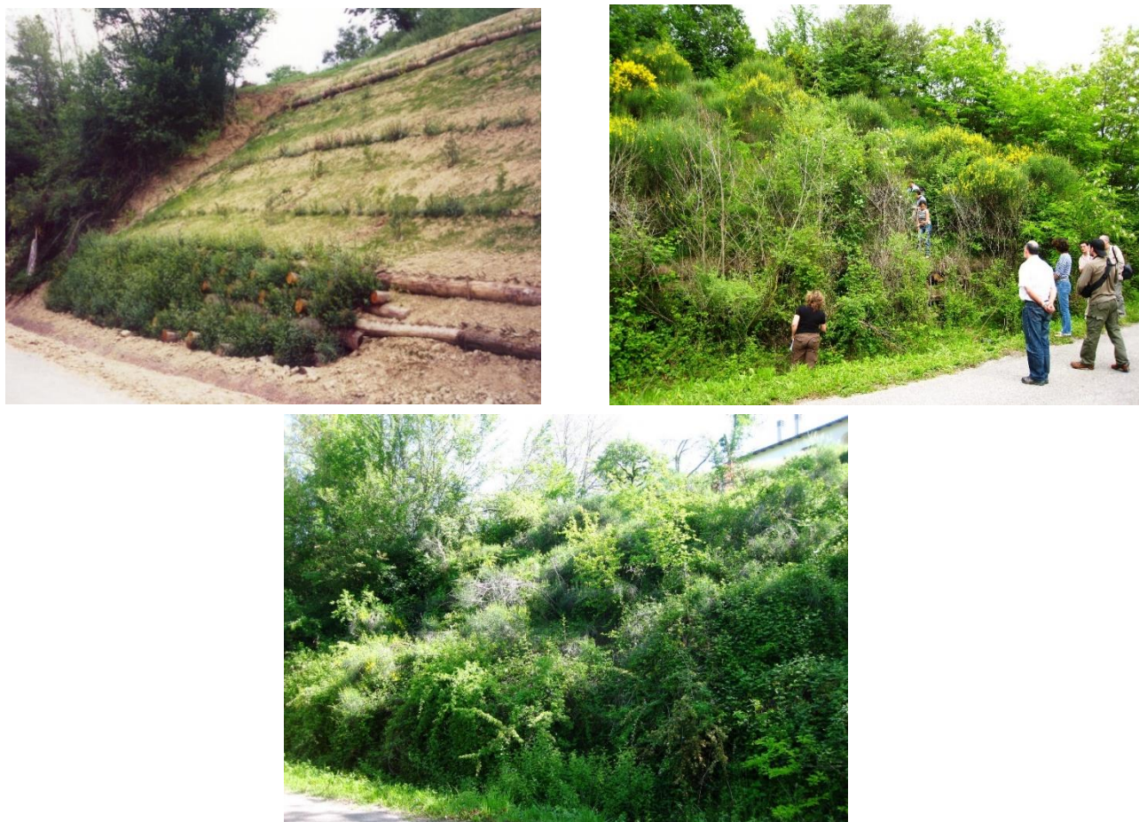
Figura 5.9 Palificata Colle Melfa (FR). 2000, 2008 e 2012.
