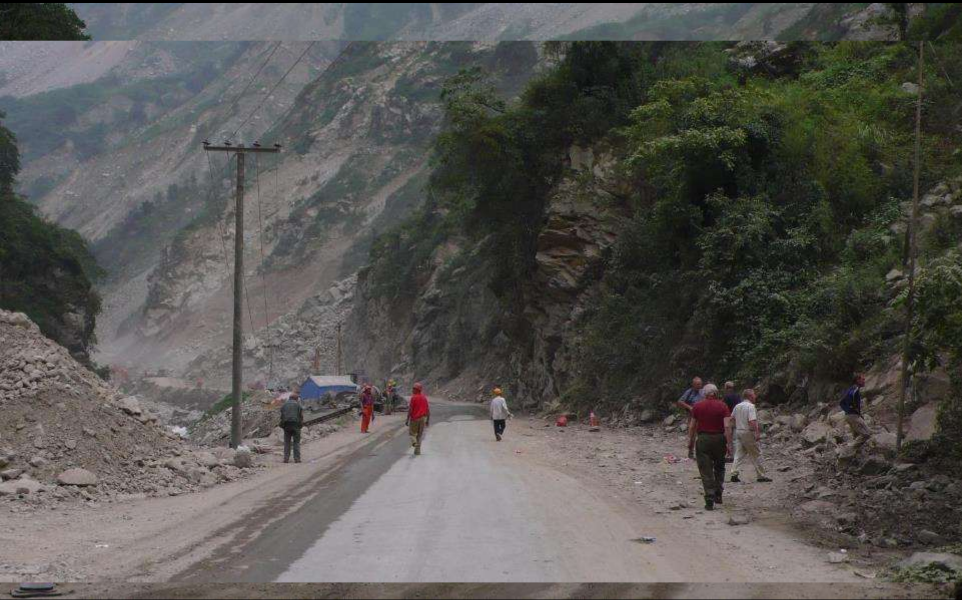
Road through the Wolong Nature reserve after the tragic Great Wenchuan earth quake of 2008
