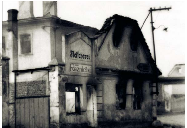
The burned-out butcher shop of Mrs. Marie Houbová that used to stand across from the church. Its last "customers" were the members of the Schupo who looted the store after their "work" in Lidice was completed, looking for snacks and refreshments. The store's owner never had the chance to learn this.
