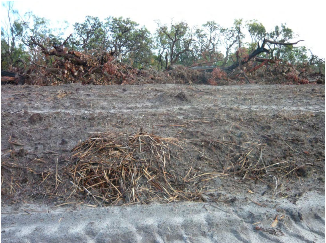
Plate 1 Topsoil and vegetation stockpiles
