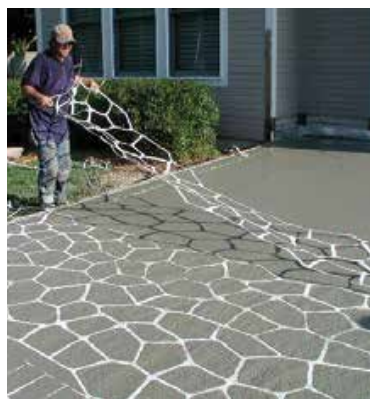
BRICK HEADER *B BRICK SIZE: 3 1/4" X 7 1/2" ROLL WIDTH: 8 1/2" JOINT WIDTH: 1/2"
