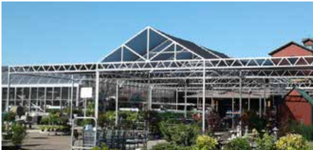
Peaked Roof W-Truss
