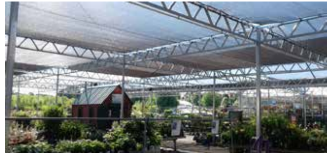
Standard Roof W-Truss
