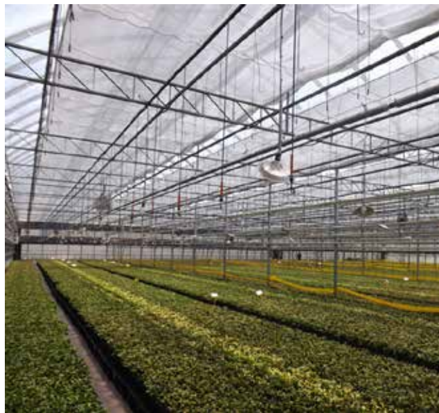
Gutter to Gutter System
