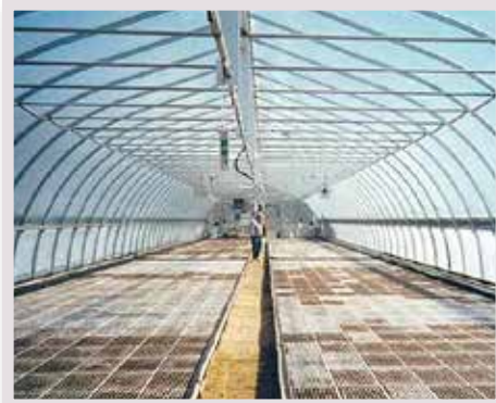
DeCloet 30ft Ground to Ground with Optional Cross Ties
