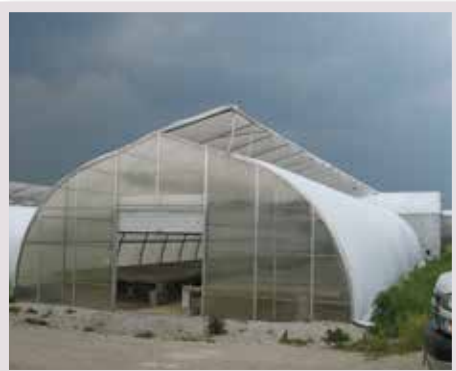
DeCloet 30ft Web Truss House with Roof Vent
