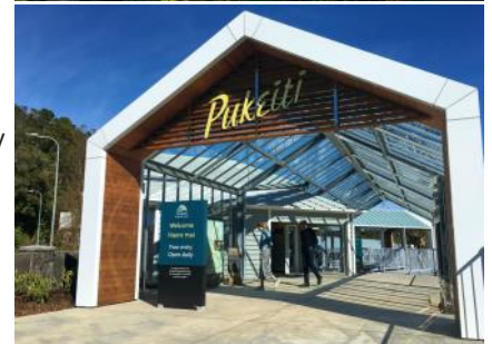
TOP & ABOVE: New entrance
