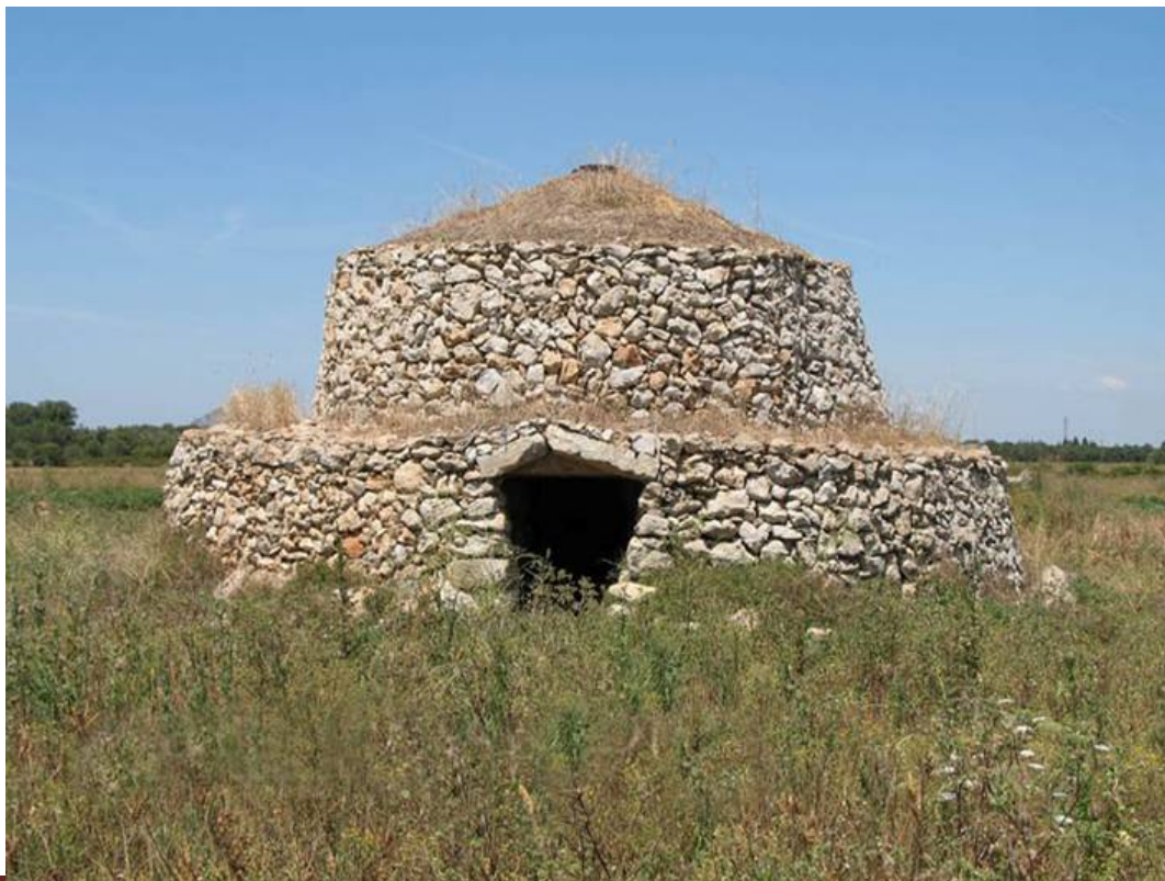
Fig. 2 – Typical dry stone shelter ( pajara )
