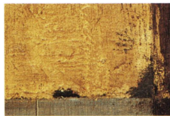
14. Detail of the Virgin and St. John panel, showing a surviving patch, above the coping stone of the wall at the right edge, of the blue background paint largely removed from the panels in 1941.
