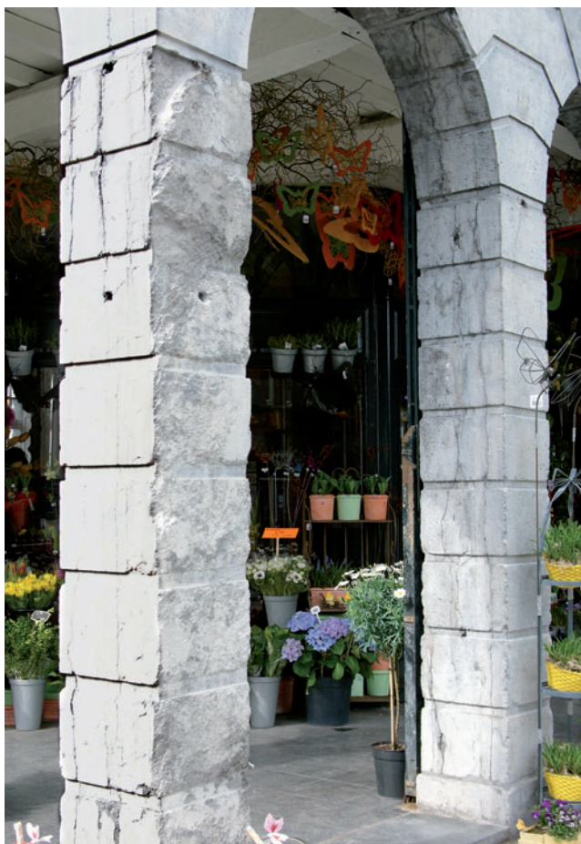
Fig. 12. Namur limestone columns of the portal of the Sentry House, built in 1786.
