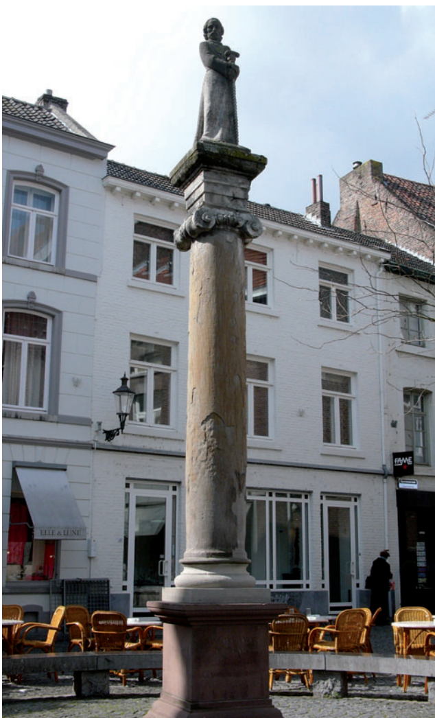
Fig. 15 St Amor statue; column of micaceous sandstone on a pedestal of Red Bunter sandstone.
