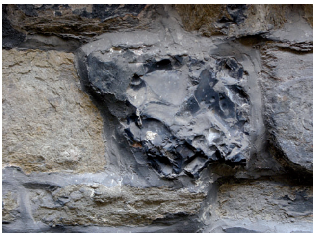
Fig. 9. Flint from the Maastricht Formation in the plinth of the Franciscan church.
