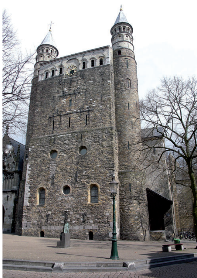
Fig. 11. Basilica of Our Beloved Lady: Maastricht limestone on top of Carboniferous sandstone and large blocks of Namur limestone.
