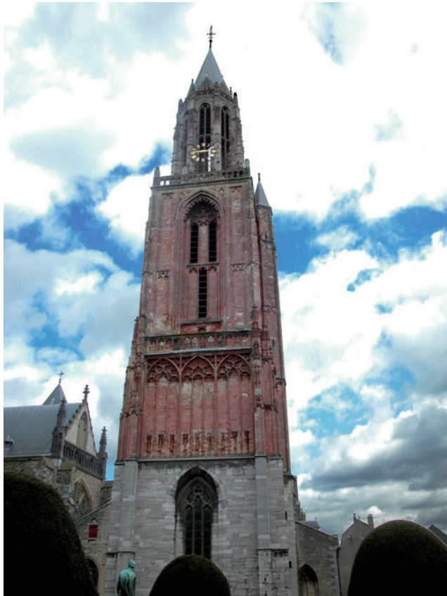
Fig. 19. Red-painted Maastricht limestone above grey Namur limestone in the tower of St John’s Church.
