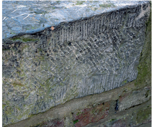
Fig. 7. Stonemason's chisel marks on Namur limestone slab. Bridge to the old mill at the River Jeker.
