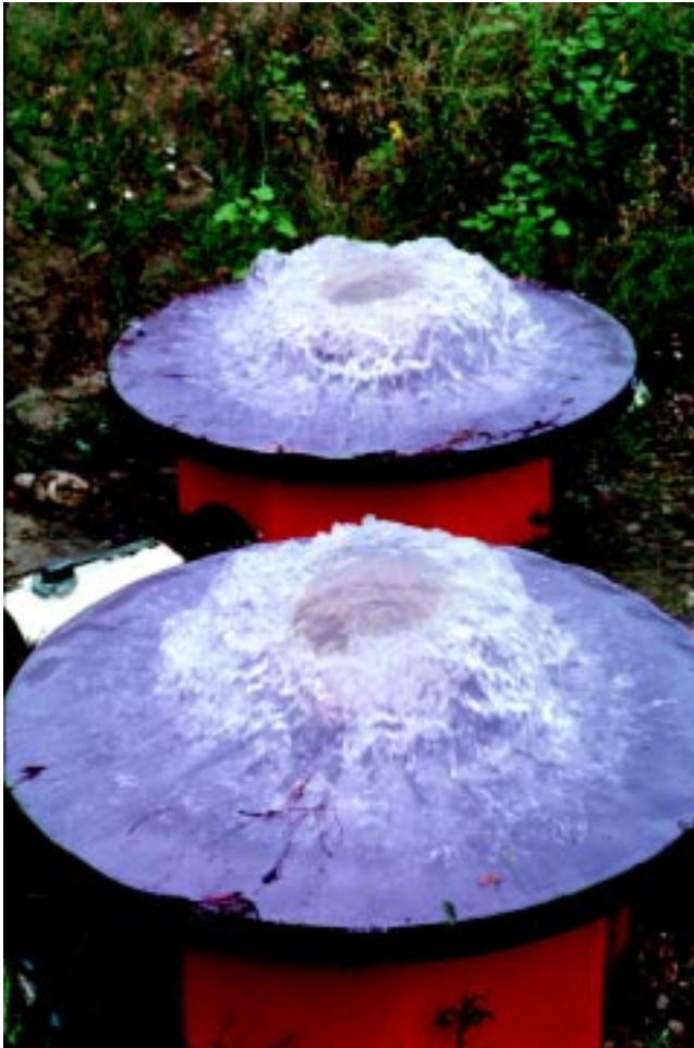
Figure 5.1. Use of self-cleaning weed screens in an irrigation system to prevent the spread of weed seeds along irrigation ditches. Photo courtesy of T. D. Whitson, University of Wyoming.
