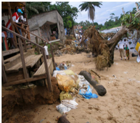
Plate 3.18-3.19: Coastal Erosion Kribi Source:– Photo by Thomas Tata (2012) but at the same time biodiversity resources can reduce the impacts of climate change on population and ecosystems.
