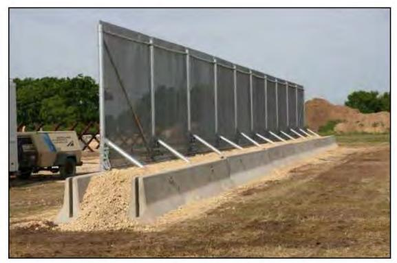
Figure E-9. Vehicle Barrier with Pedestrian Fence
