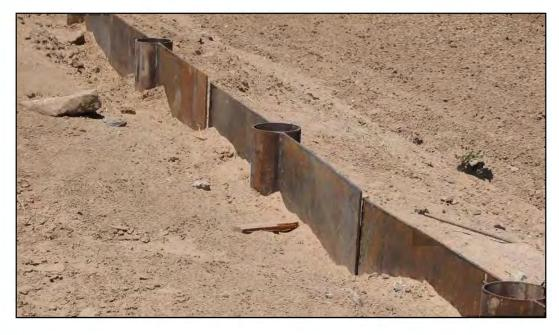
Figure E-1. Typical Pedestrian Fence Foundation
