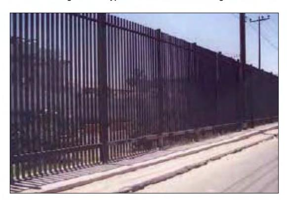
Figure E-4. Typical Pedestrian Fence Design
