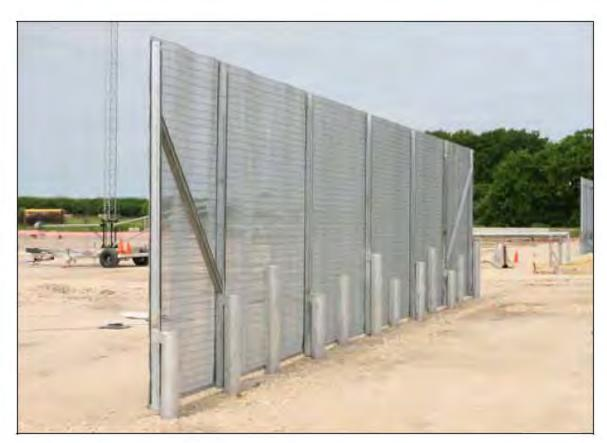
Figure E-8. Vehicle Barrier with Pedestrian Fence
