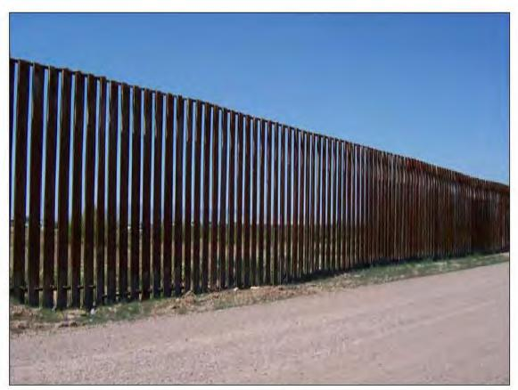
Figure E-10. Bollard Fence
