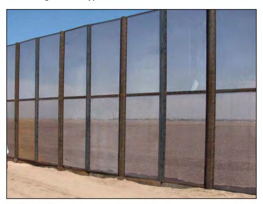
Figure E-2. Typical Pedestrian Fence Design
