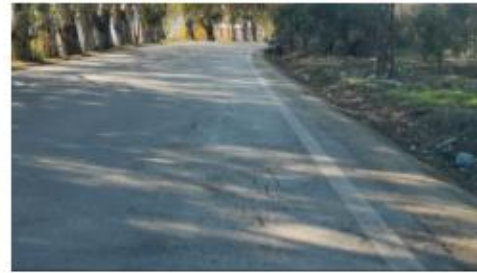
Obstructed channels and damaged pavement
