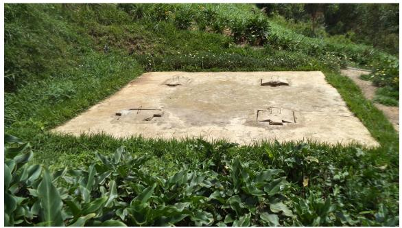
Photo 5: New wastewater treatment system installed by Teza tea factory, preventing the pollution of the Nyabihondo River.
