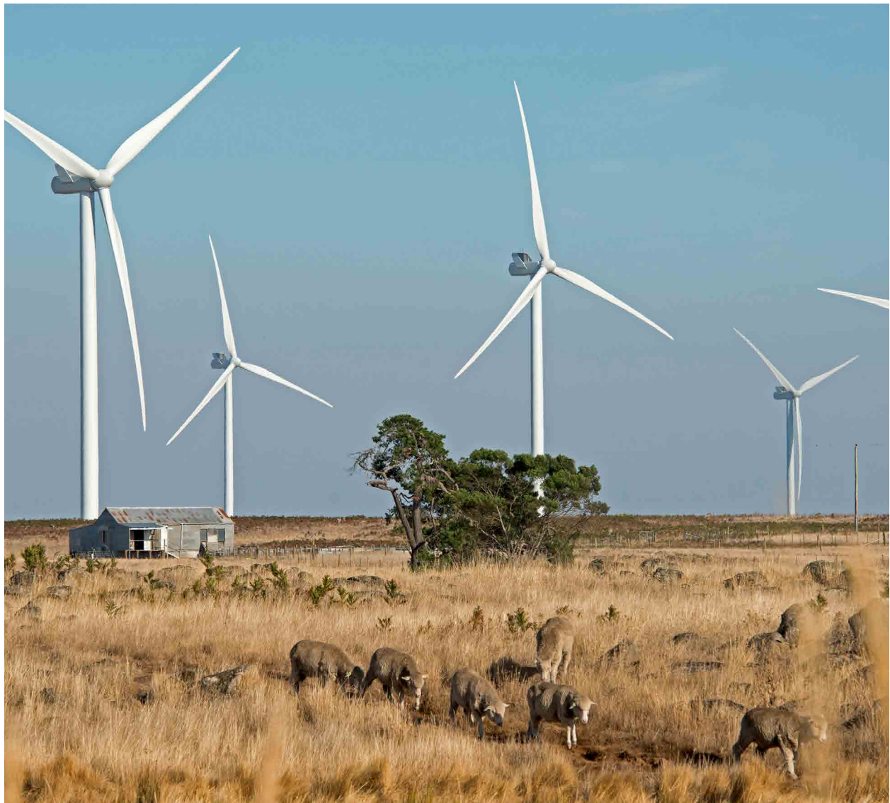
Wind farm near Hamilton, Victoria.
