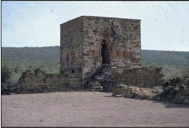
Example of a Fortified Structure (Fort Double Drift)
