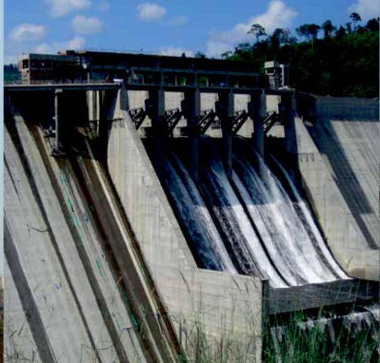
Kamchay Hydropower Plant in Kampot Province
