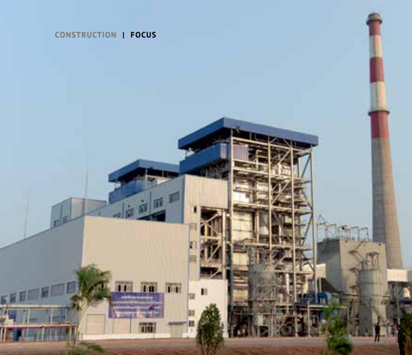
Coal-fired power plant 100MW in Preah Sihanouk Province
