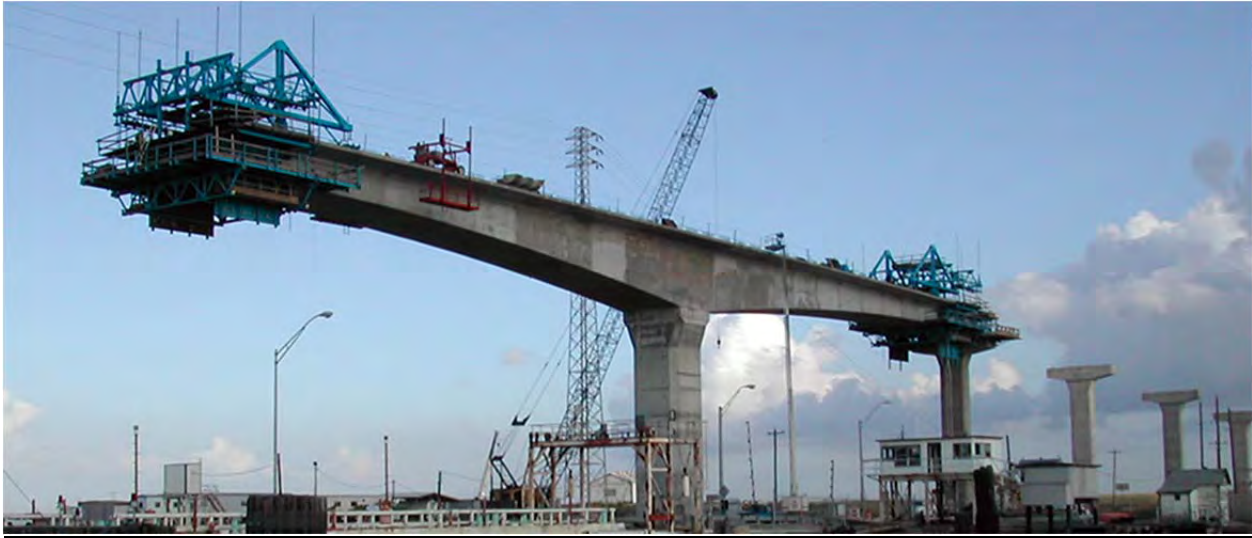
FIGURE 3 - PRECAST SEGMENTAL CONCRETE
