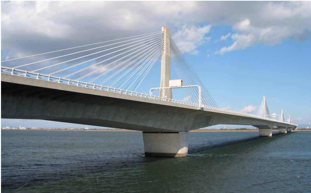
FIGURE 7 - EXTRADOSED PRECAST SEGMENTAL CONCRETE
