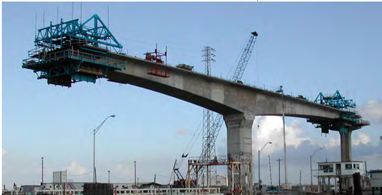
Figure 7: Precast Segmental Concrete Spans
