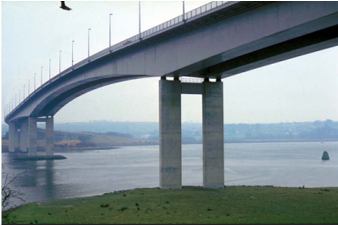
FIGURE 6 - TRAPEZOIDAL STEEL BOX GIRDERS
