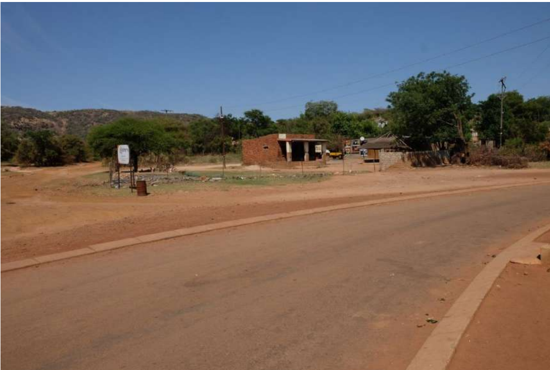
Photo 2: Photo showing the typical condition of the existing access road
