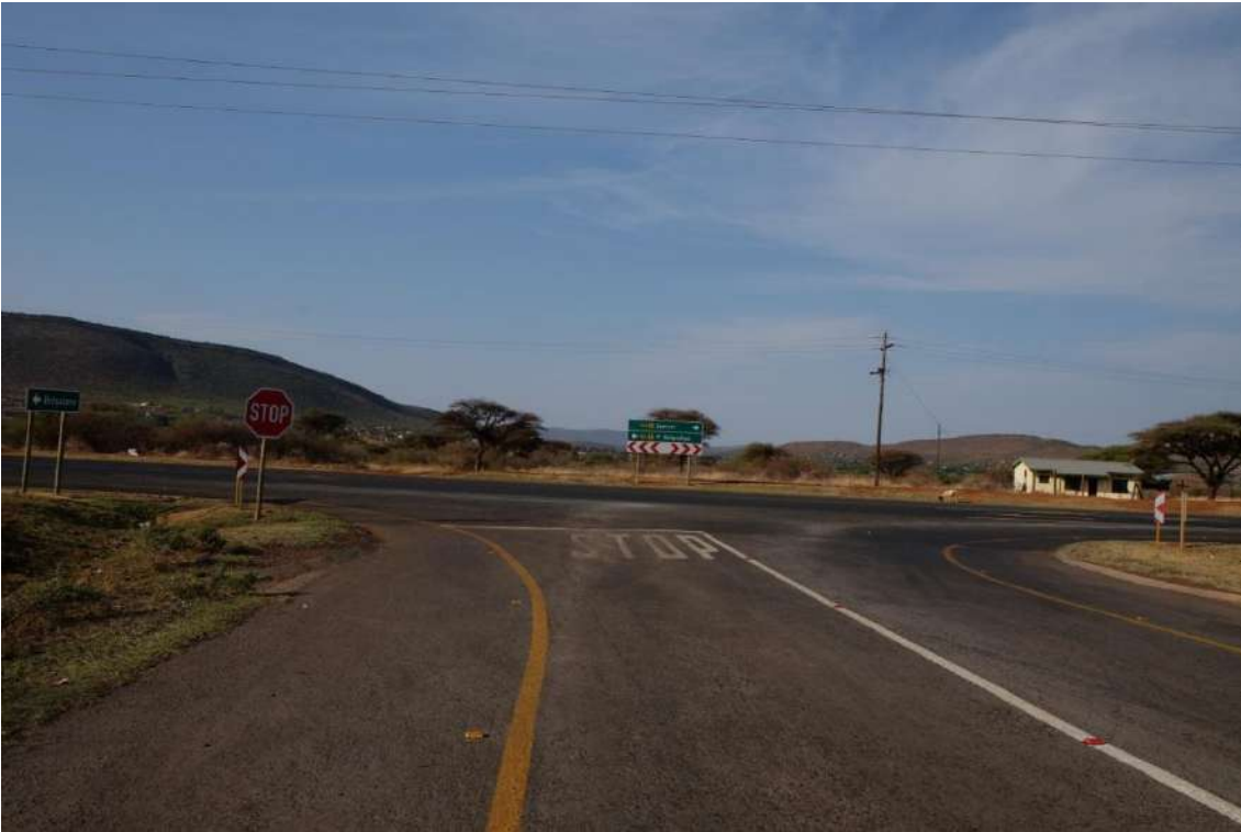
Photo 3: T-intersection of the access road and the N4, taken in an northern direction
