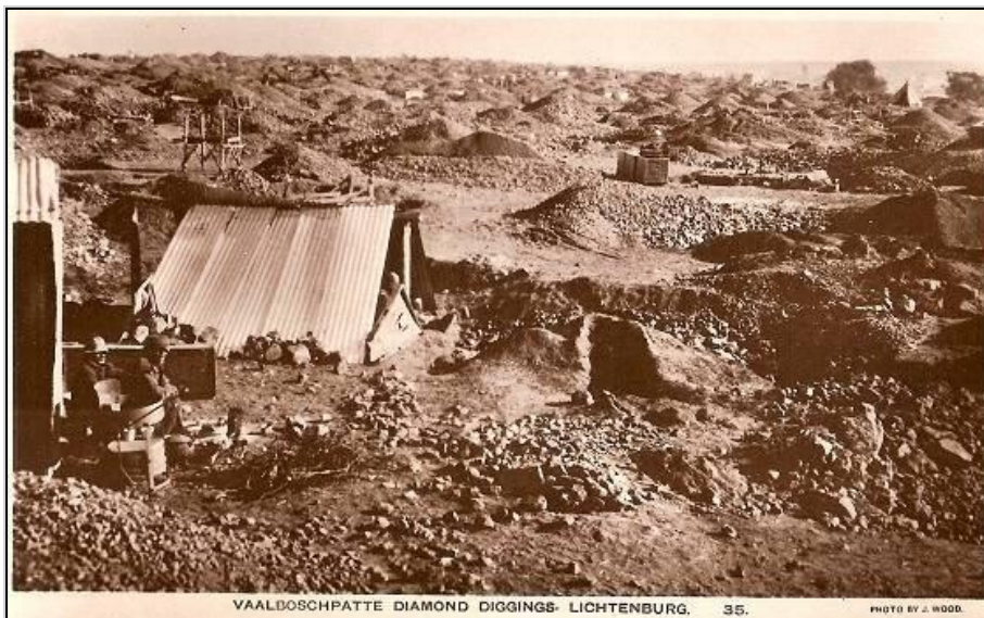
Figure 1-8: Vaalboschpatte Diamond Diggings (Source: Smith 2006).
