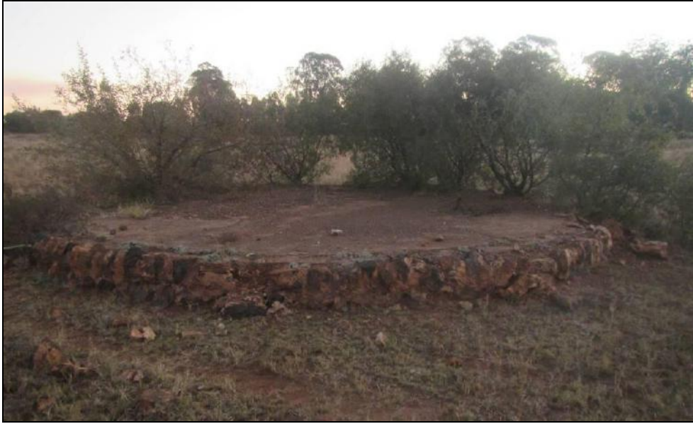
Figure 10: The circular foundation found at waypoint 167.
