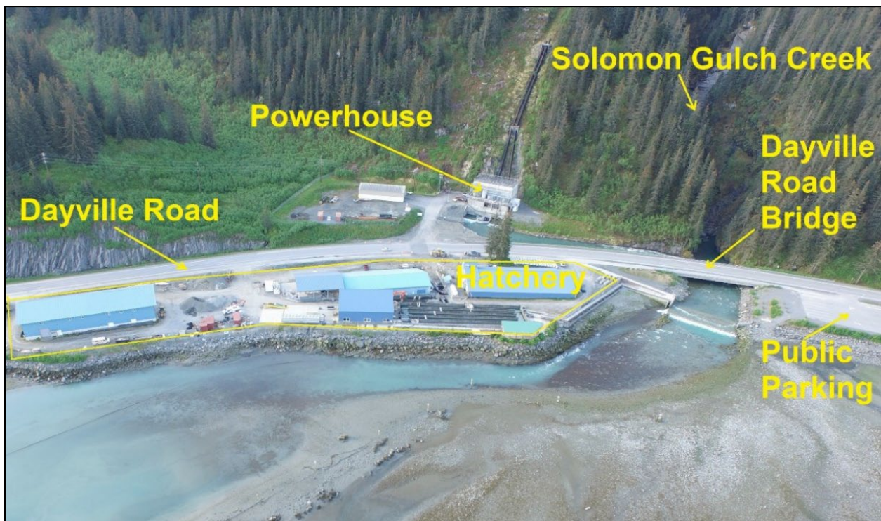
Photo 5-5 Solomon Gulch Hydroelectric Powerhouse and Tailrace, Solomon Gulch Hatchery, and the Mouth of Solomon Gulch Creek
