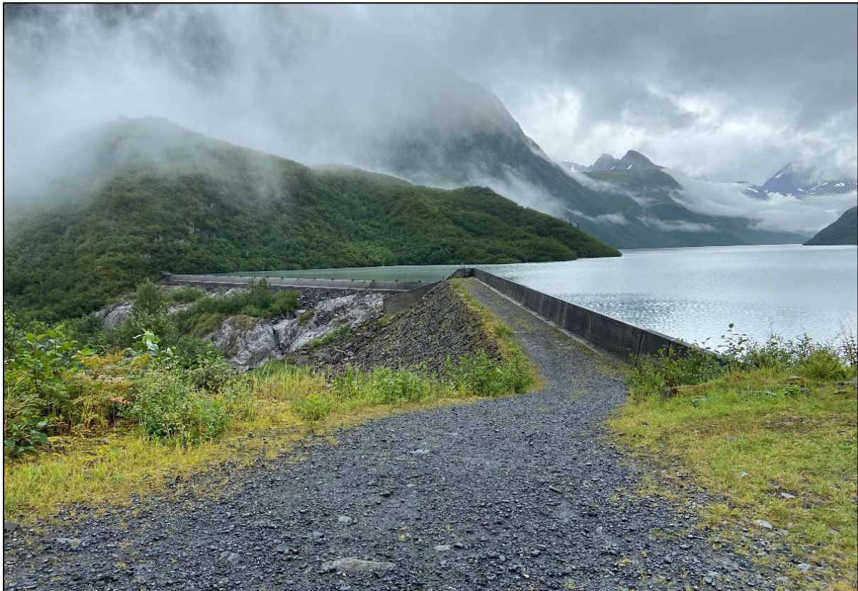
Photo 5-13 Concrete Spillway and Rockfill Embankment Dam
