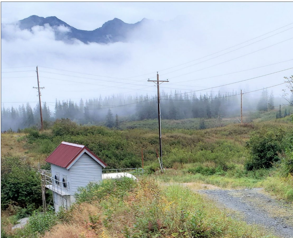
Photo 3-5 Solomon Gulch Project Low Level Outlet Works
