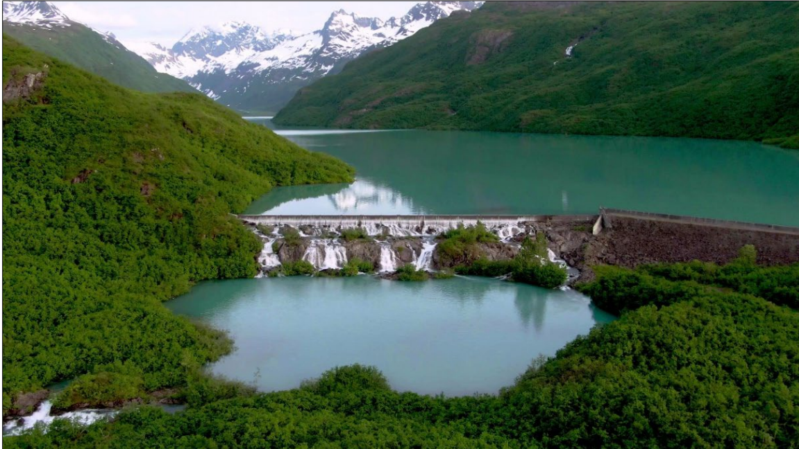
Photo 3-3 Solomon Gulch Project Spillway and Saddle Dike
