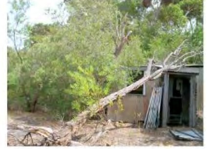
Derelict shed below Minsterly Road
