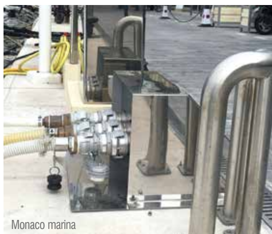
Polished mirror stainless steel cabinet with black water sewer
