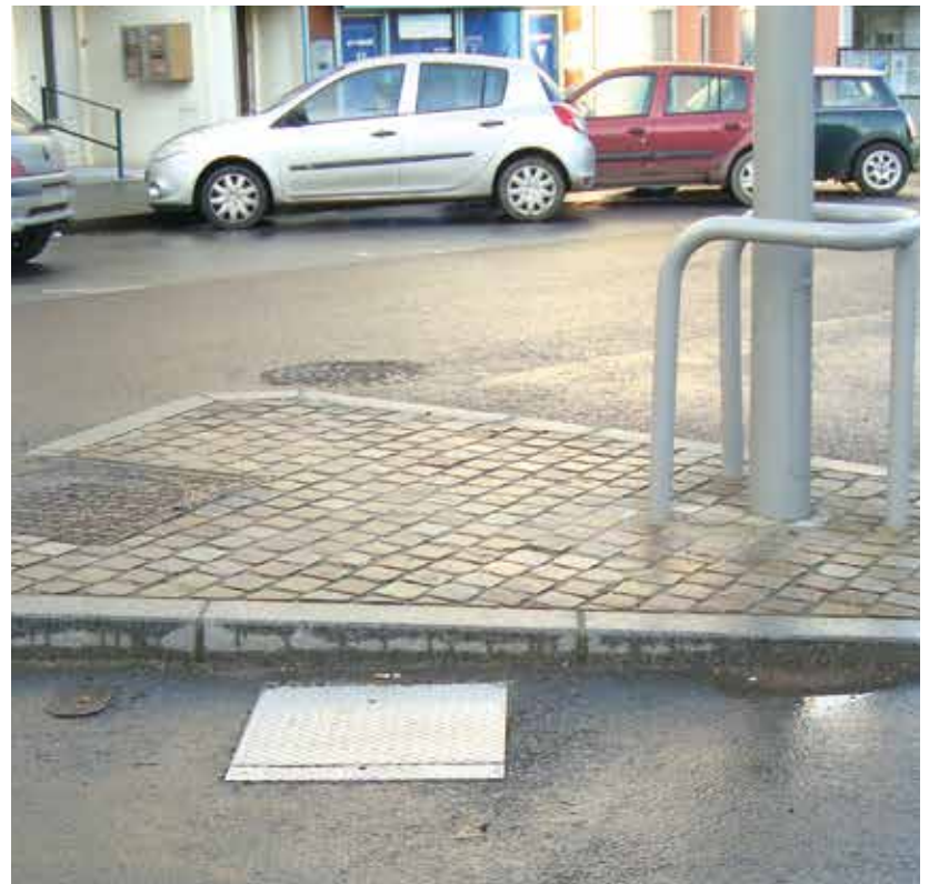
Retractable Sourcinox pedestal 06 in closed position, Saint-Lô
