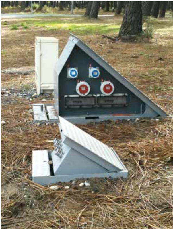
Retractable Sourcinox pedestals 01 and 10 in the open position, La-Teste-de-Buch
