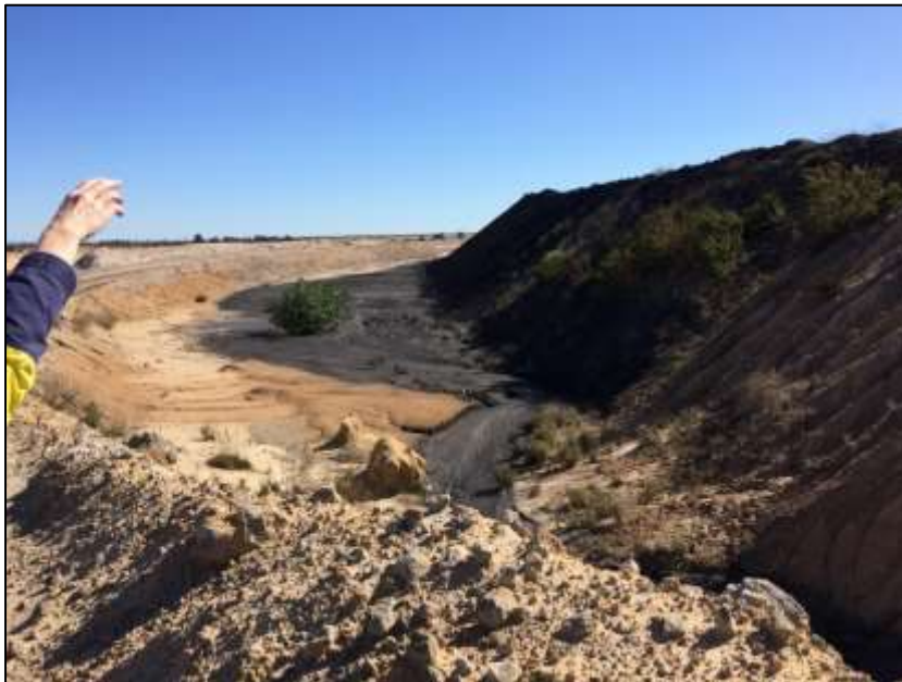
Figure 13: Seepage and surface water runoff from the MRF is contained within the perimeter embankment area.
