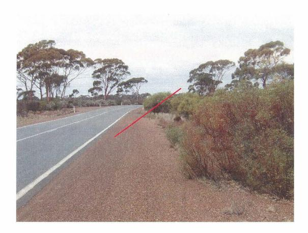
Possible realignment required on inside of curve to improve horizontal geometry. Red line indicates approximate area required for realignment.
