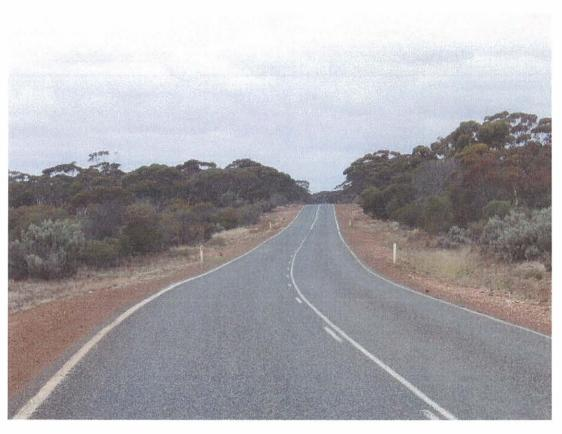
Photo Emu Rocks to Widgiemooltha Project looking south along the Great Eastern Highway. Existing seal width approximately 7m. Planned seal width 8m on 10m wide formation Guide Post shown in photo are approx 9.8m
