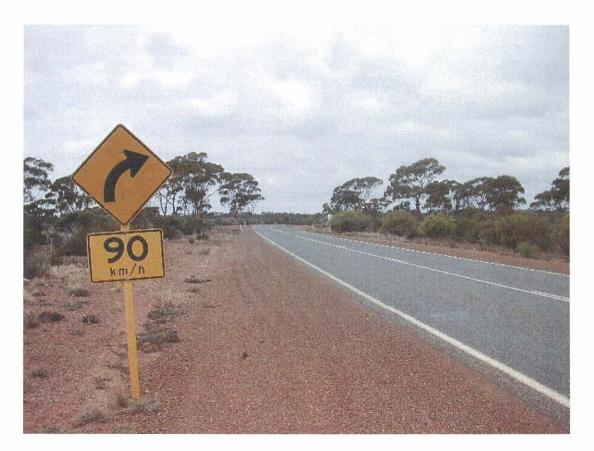
Possible realignment (minor) required on this cure to improve horizontal geometry
