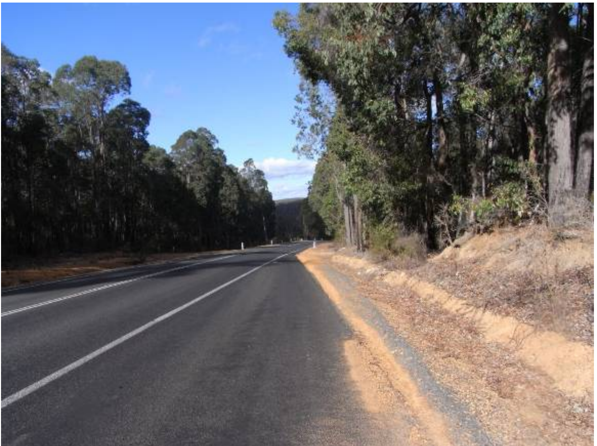
Photo 5: View east SLK 27.65 – Start of existing passing bay and 70m west of the eastern extent of the project.
