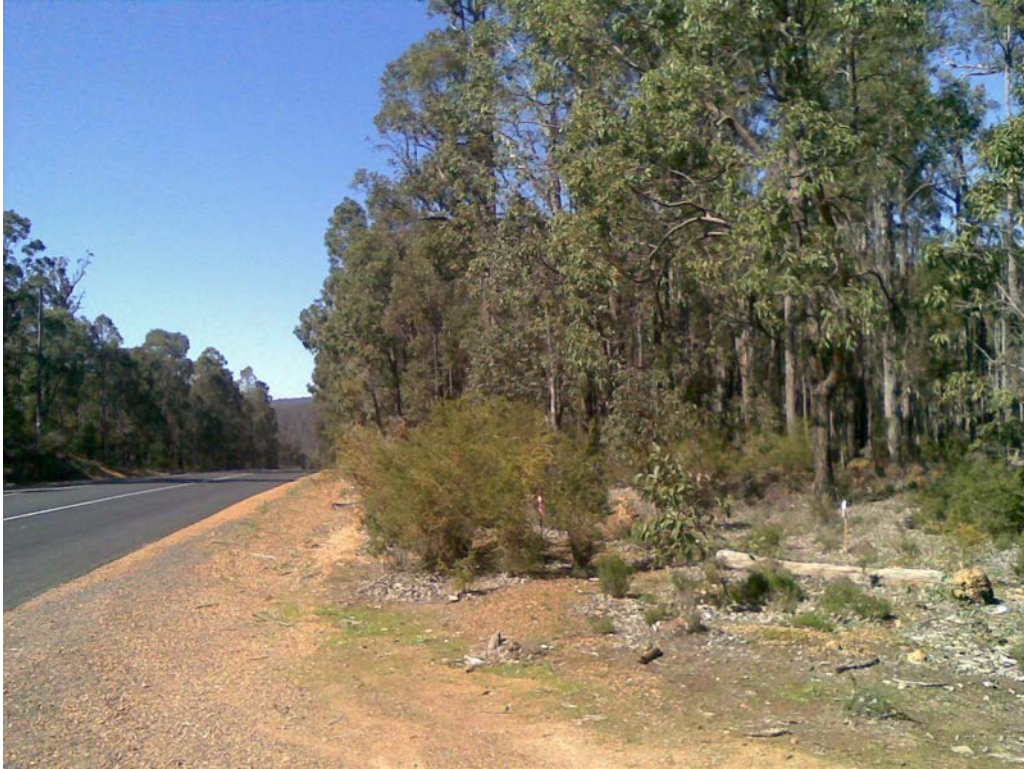
Photo 2: View east SLK 27.54 – inside peg is road reserve boundary, outside peg is the ideal lateral clearance.
