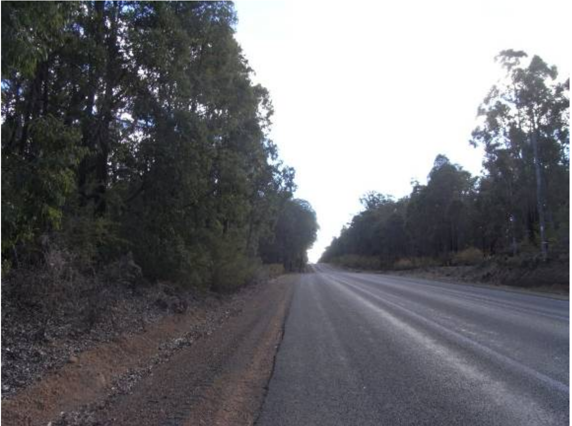
Photo 4: View west SLK 27.65 – Existing passing bay indicating width of clearing required.
